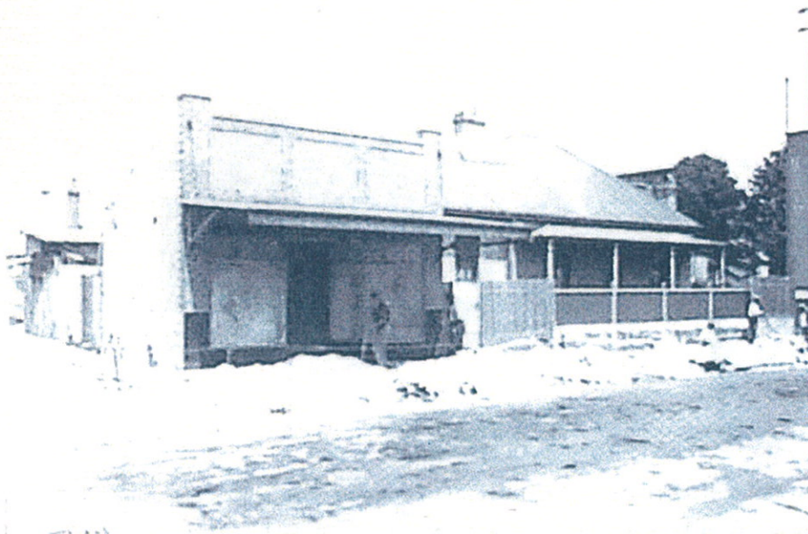
Figure 2.9 Front view of 4-6 Pitt Street before demolition, 1926
